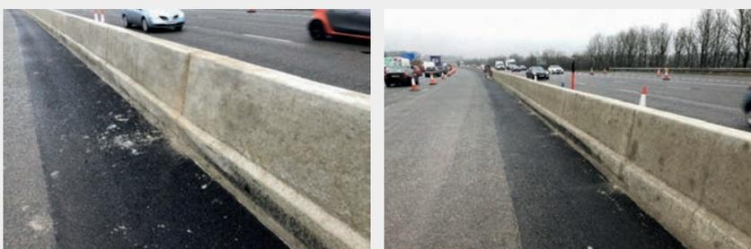
**On Friday 9th March 2018, a serious breach of traffic management was encountered on the M62 J30 to 31 scheme when an HGV collided with newly installed Concrete Barrier. The incident had the potential to result in significant injury or even fatality.**
